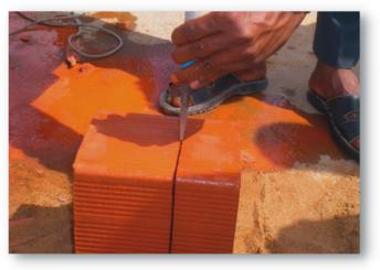
Step: 2 Cut along the marked area using the wet cutter
